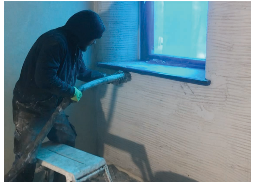
Pump applied hemp plaster
